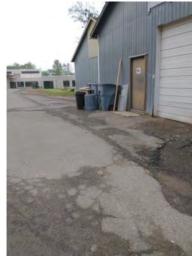
Photograph 8: View of Maintenance Pavement Area.
