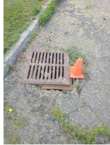
Photograph 6: View of storm drain located at the Parking Lot Pavement Area.
