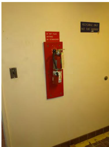
Photograph 3: View of fire extinguisher in room no. 5C32.
