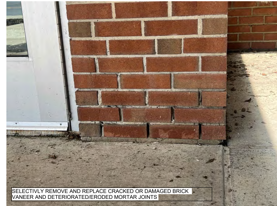
SELECTIVELY REMOVE AND REPLACE CRACKED OR DAMAGED BRICK VANEER AND DETERIORATED/ERODED MORTAR JOINTS
