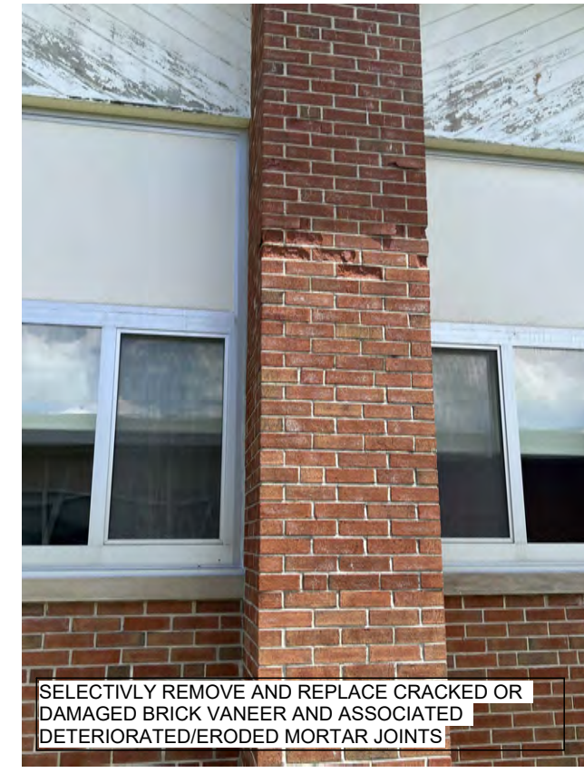
SELECTIVELY REMOVE AND REPLACE CRACKED OR DAMAGED BRICK VANEER AND ASSOCIATED DETERIORATED/ERODED MORTAR JOINTS
