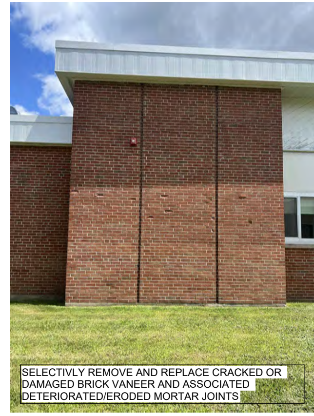
SELECTIVELY REMOVE AND REPLACE CRACKED OR DAMAGED BRICK VANEER AND ASSOCIATED DETERIORATED/ERODED MORTAR JOINTS
