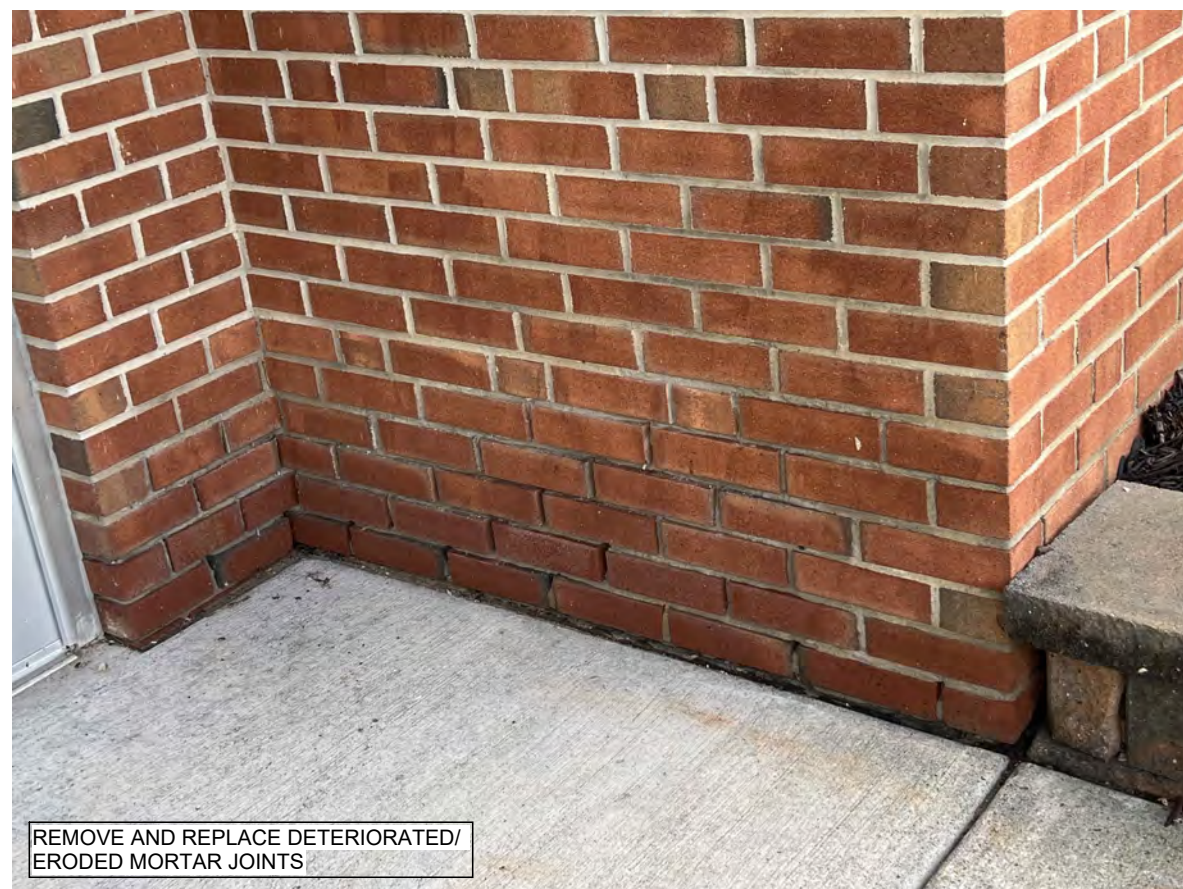
13 BRICK FACADE REPAIR SCALE: 3/32" = 1'-0"
