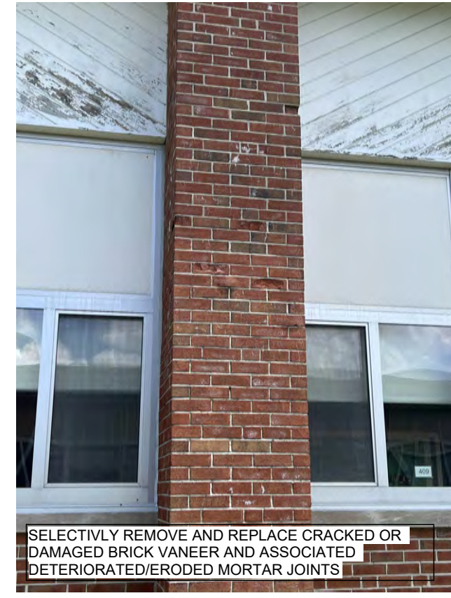
SELECTIVELY REMOVE AND REPLACE CRACKED OR DAMAGED BRICK VANEER AND ASSOCIATED DETERIORATED/ERODED MORTAR JOINTS
