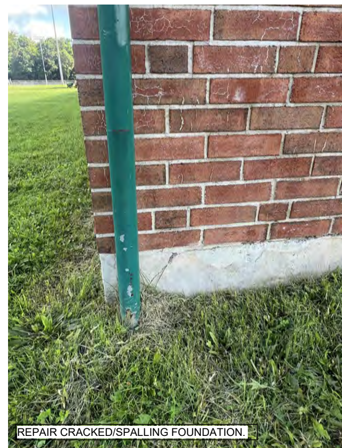
14 FOUNDATION REPAIR SCALE: 3/32" = 1'-0"
