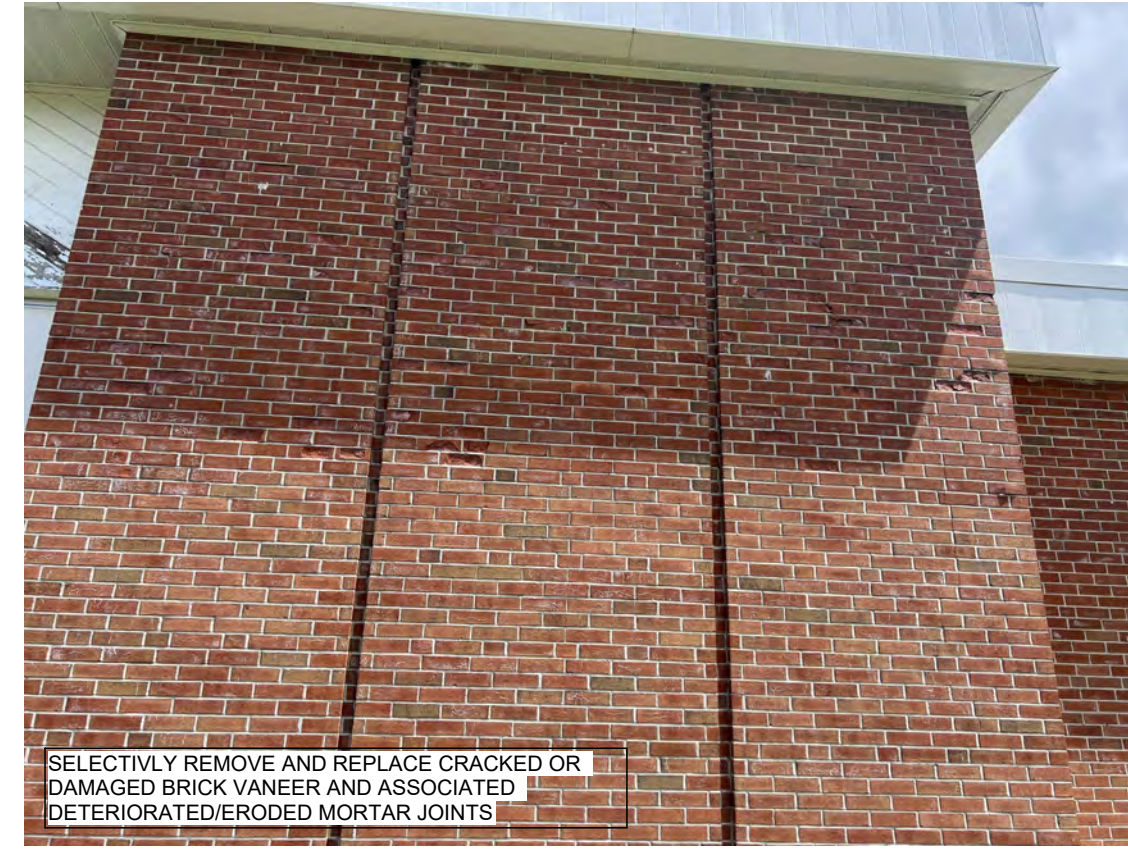
SELECTIVELY REMOVE AND REPLACE CRACKED OR DAMAGED BRICK VANEER AND ASSOCIATED DETERIORATED/ERODED MORTAR JOINTS
