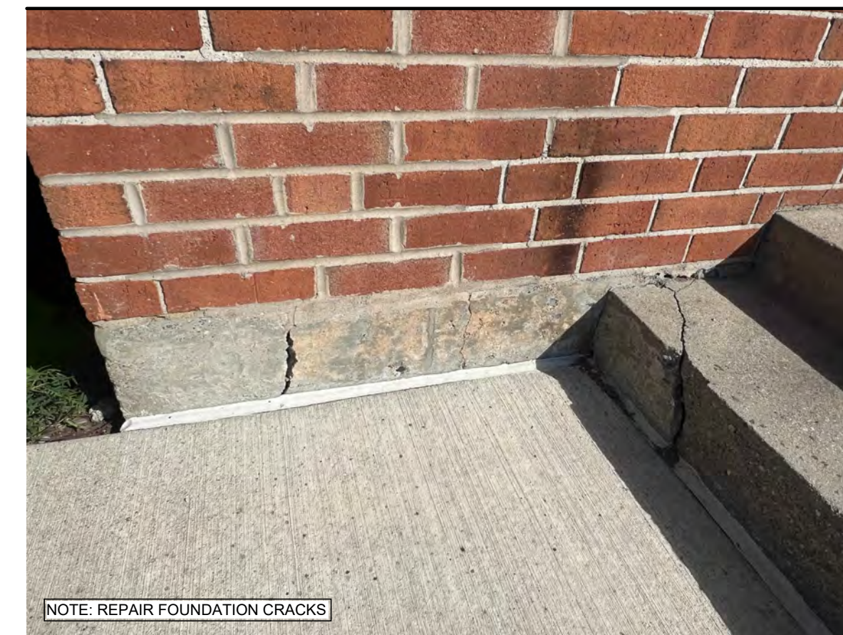
1 FOUNDATION REPAIR SCALE: NTS
