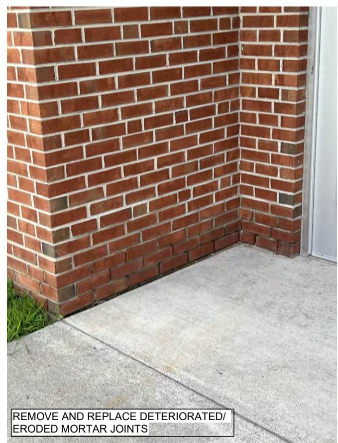
17 BRICK FACADE REPAIR SCALE: 3/32" = 1'-0"
