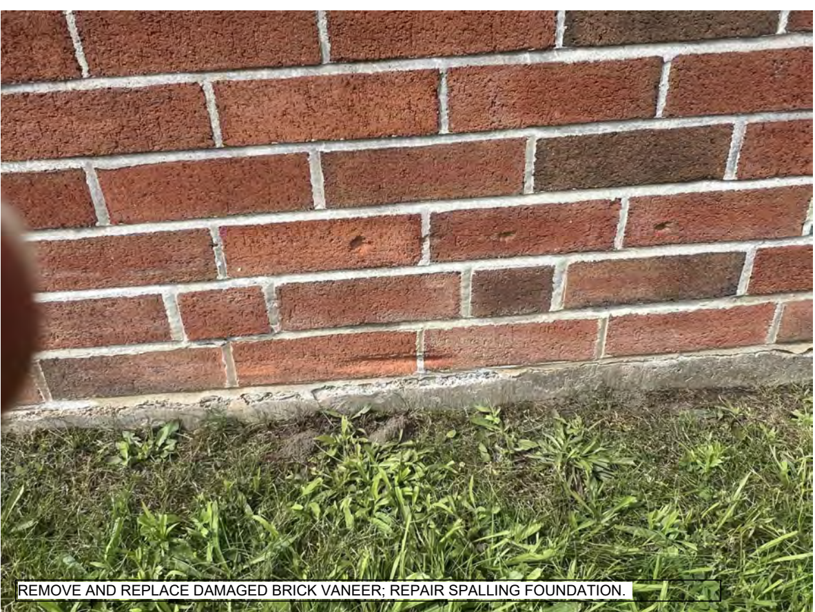
11 FOUNDATION AND FACADE REPAIR SCALE: 3/32" = 1'-0"
