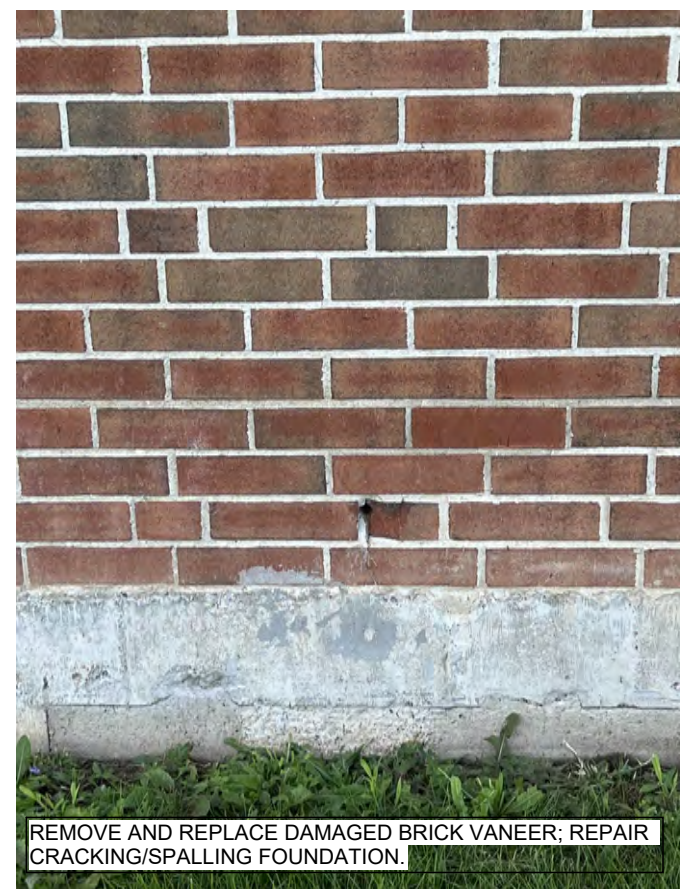
13 BRICK FACADE REPAIR SCALE: 3/32" = 1'-0"
