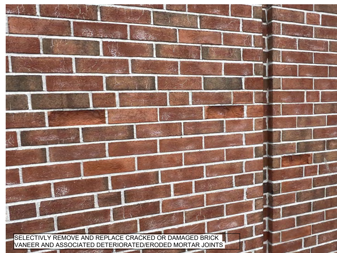
15 BRICK FACADE REPAIR SCALE: 3/32" = 1'-0"
