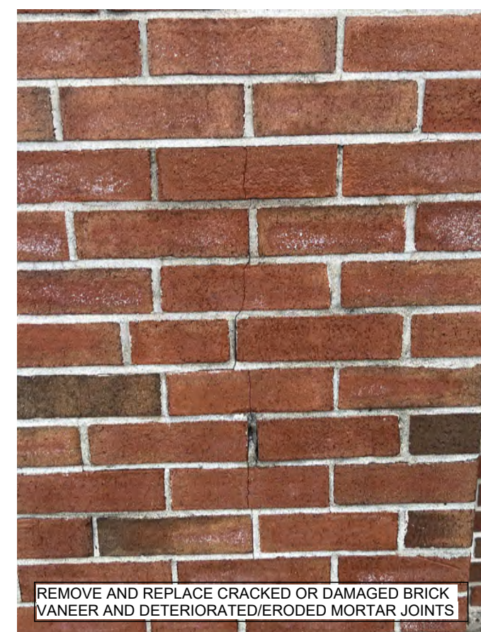
10 FACADE REPAIR SCALE: 3/32" = 1'-0"
