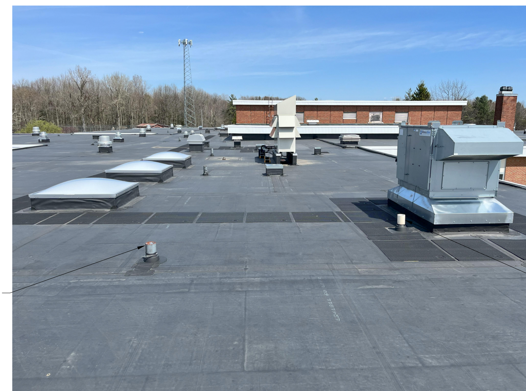
3 PICTURE OF ROOFTOP ABOVE SCALE: 1/4" = 1'-0"
