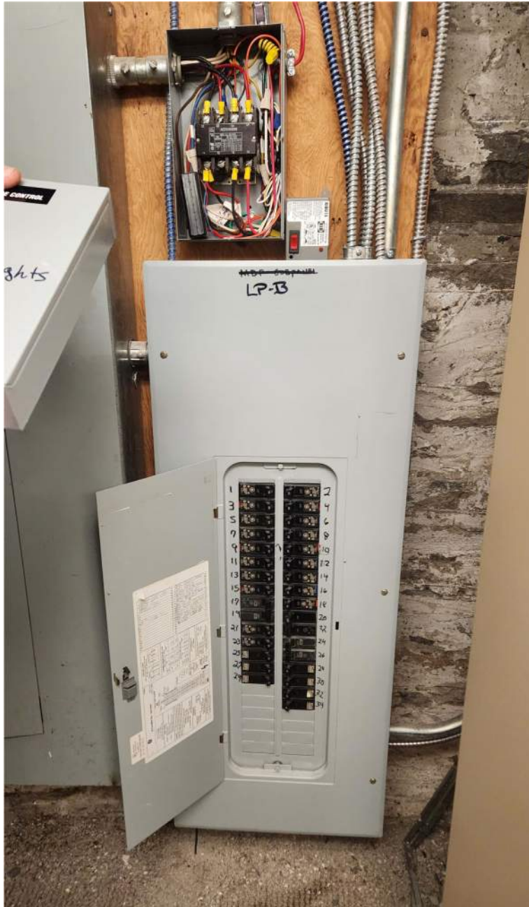
Secondary panel inside Merrill House conference room electrical closet. Secondary panel has space for additional circuits, but existing contactor is full. Contractor must provide all materials and labor to provide fully functional site lighting system.
